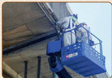
橋梁の目視点検
